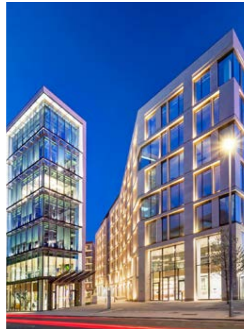
Charlemont Square Dublin - Ireland
